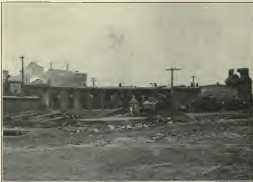
FIG. 661. FACILITIES TO BE ABANDONED. Locomotive engine house of the Illinois Central Railroad at E. 26th Street and Lake Michigan. This is a 20-stall structure built in 1898. Stalls are 75 feet long, and the construction is of the usual type with brick walls and wooden roof. Immediately to the south of this building is a second engine house having 23 stalls. In the event of electrification, this building would be rendered worthless to the railroad.
